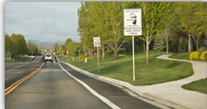
Field Application – Eagle Road, Eagle
