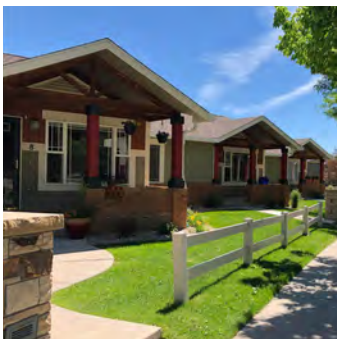
1-story, attached, single-family 4 to 8 units
