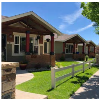
1-story, attached, single-family 4 to 8 units
