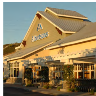
Stucco mix with pitched roofs
