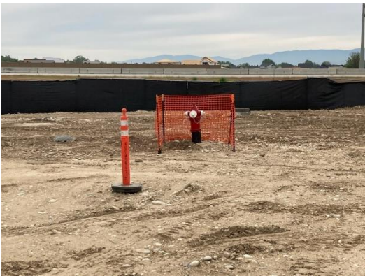
FIGURE 8-6B-3(a) HYDRANT FENCING
