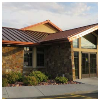
Stone siding with metal roof
