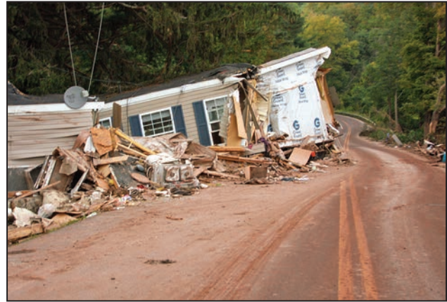
A flooded manufactured home can float off its foundation and cause additional damage nearby.
