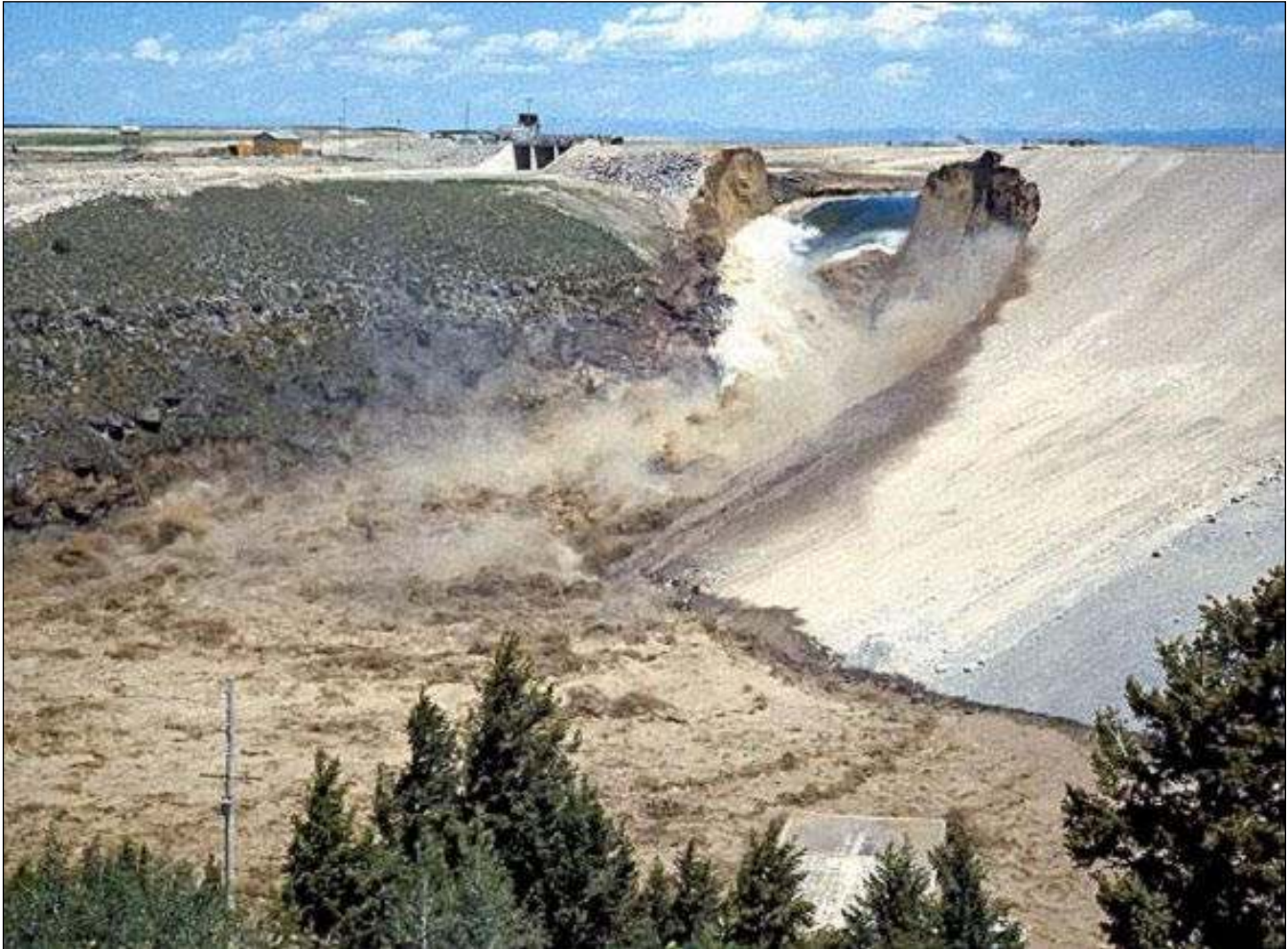
Figure 10-1. Teton Dam Failure, 1976
