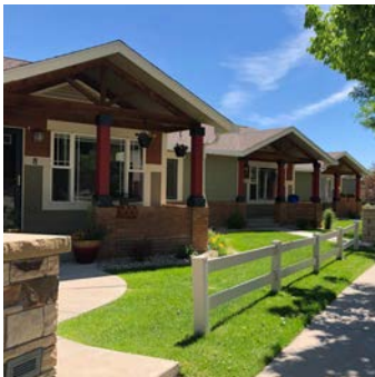
1-story, attached, single-family 4 to 8 units
