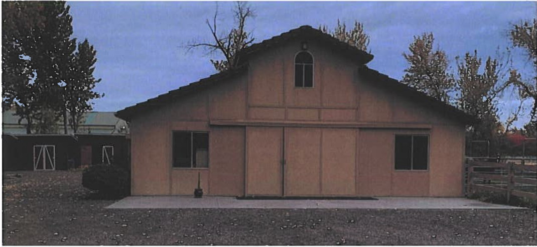
South face of existing barn.
