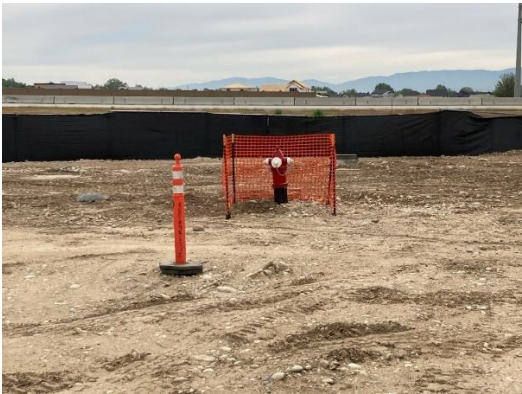
FIGURE 8-6B-3(a) HYDRANT FENCING
