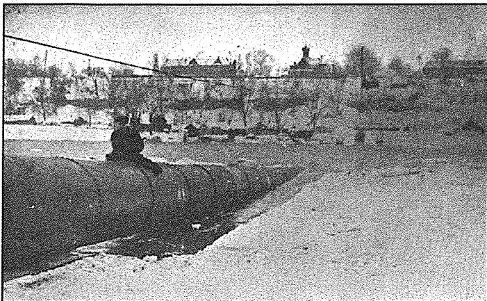
A photo from 1916 taken from the eastern bank of the Mississippi River (above) shows the construction of a trench for a waterline to be placed in the river bed. A 1917 photo (below), taken from the west bank of the river, shows the riveted steel pipe being submerged.
