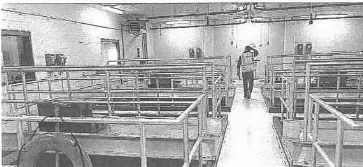
The flocculation basins and filters in Two Harbors.
