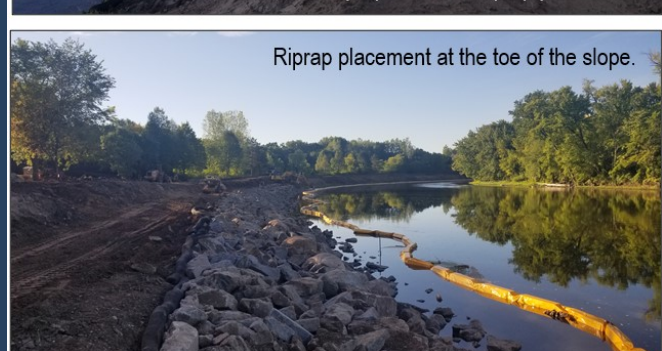
Tree clearing and bank reshaping in preparation for riprap placement.
