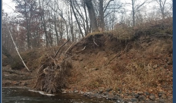
Prior Bank Condition
