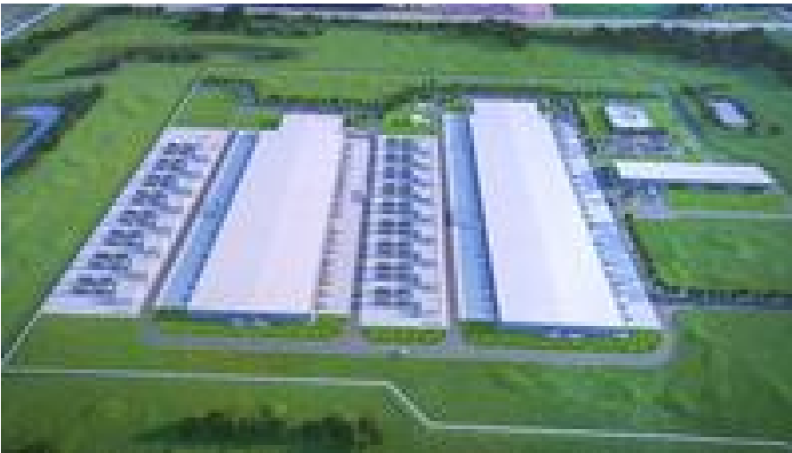
Meta to build $800M data center in Rosemount
