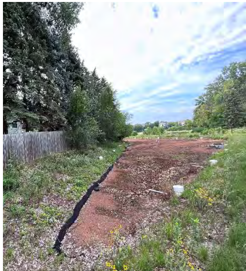
Figure 5 Golden Lake Iron Enhanced Sand Filter at Golden Lake Park in Circle Pines
