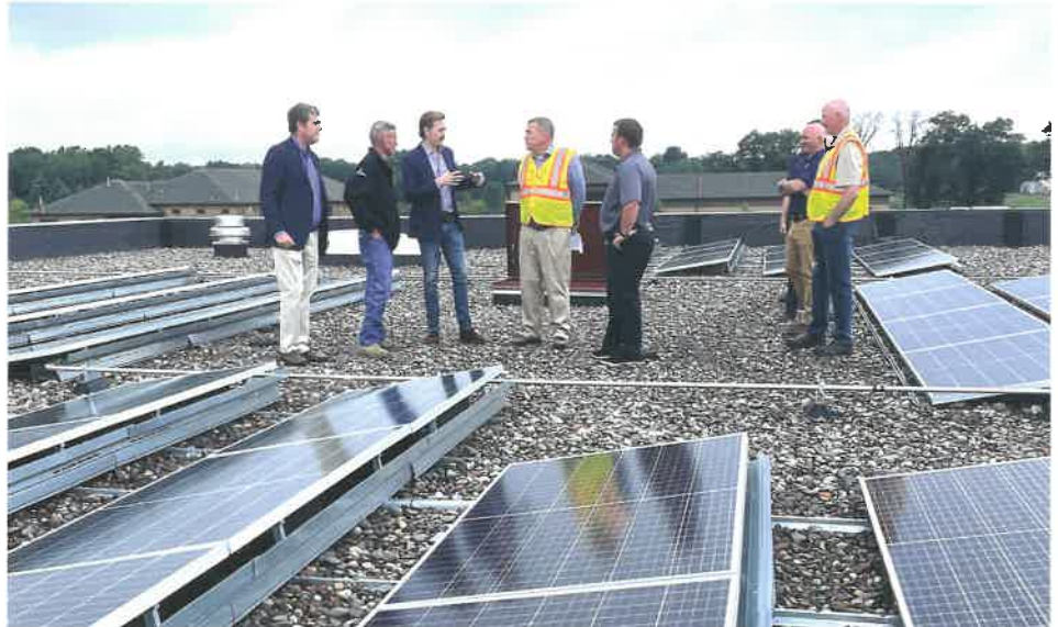
CEO Greg Ridderbush and CFO Yan Paul Martinez joined leaders from Pan-O-Gold and Ideal Energy to tour a newly installed rooftop solar array at Pan-O-Gold's new distribution warehouse in East Bethel.
