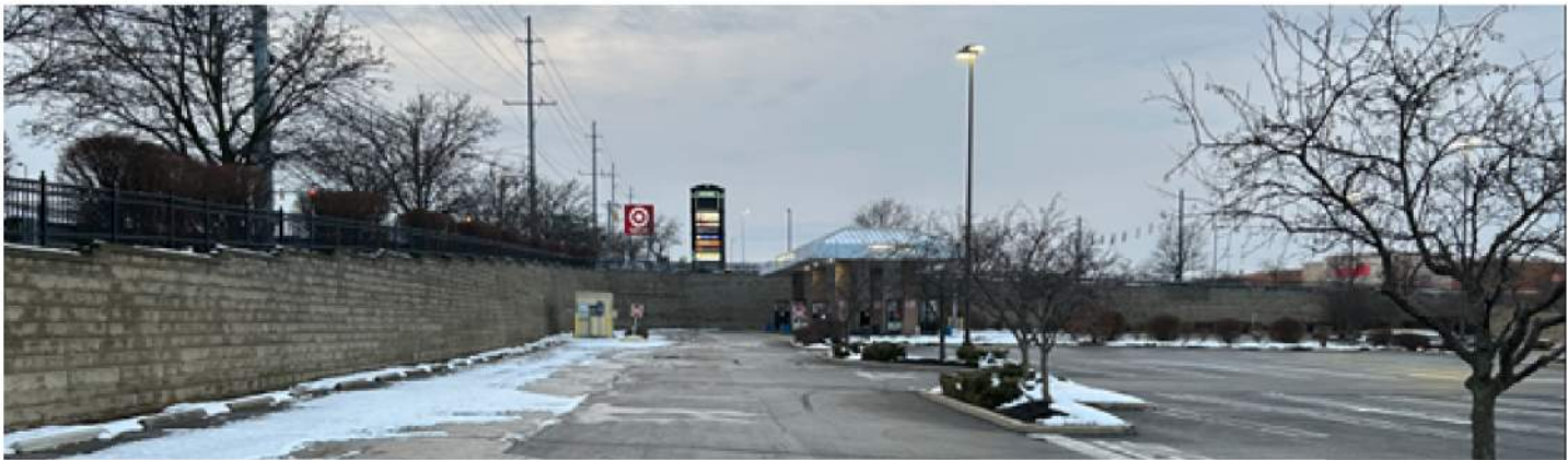
View of retaining wall at the corner of East Kemper Road and Commons Drive, screening existing Fueling Station
