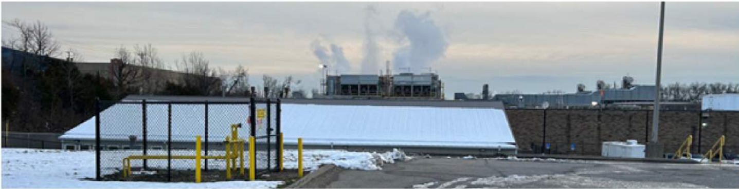
Nearby John Morrell (mechanical equipment very visible)
