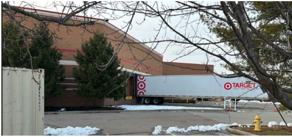
Loading Docks at Target
