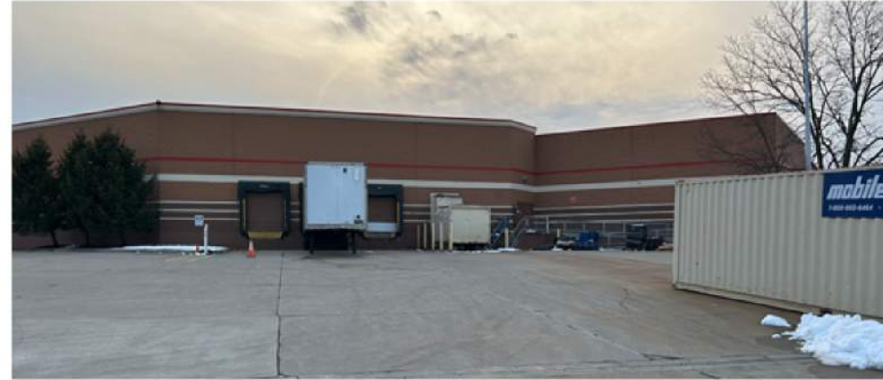
Loading Docks at Target
