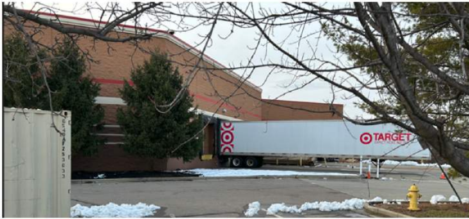
Loading Docks at Target
