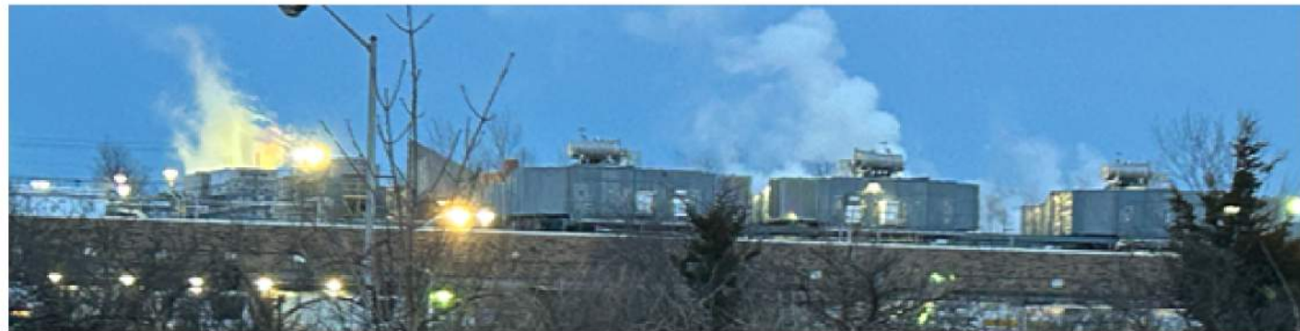
Nearby John Morrell (mechanical equipment very visible)
