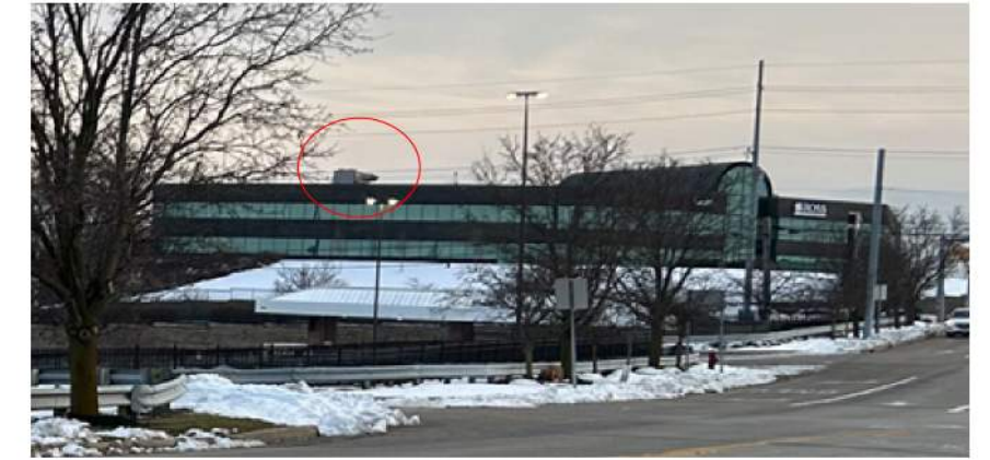
RTUs visible on Office building to the south
