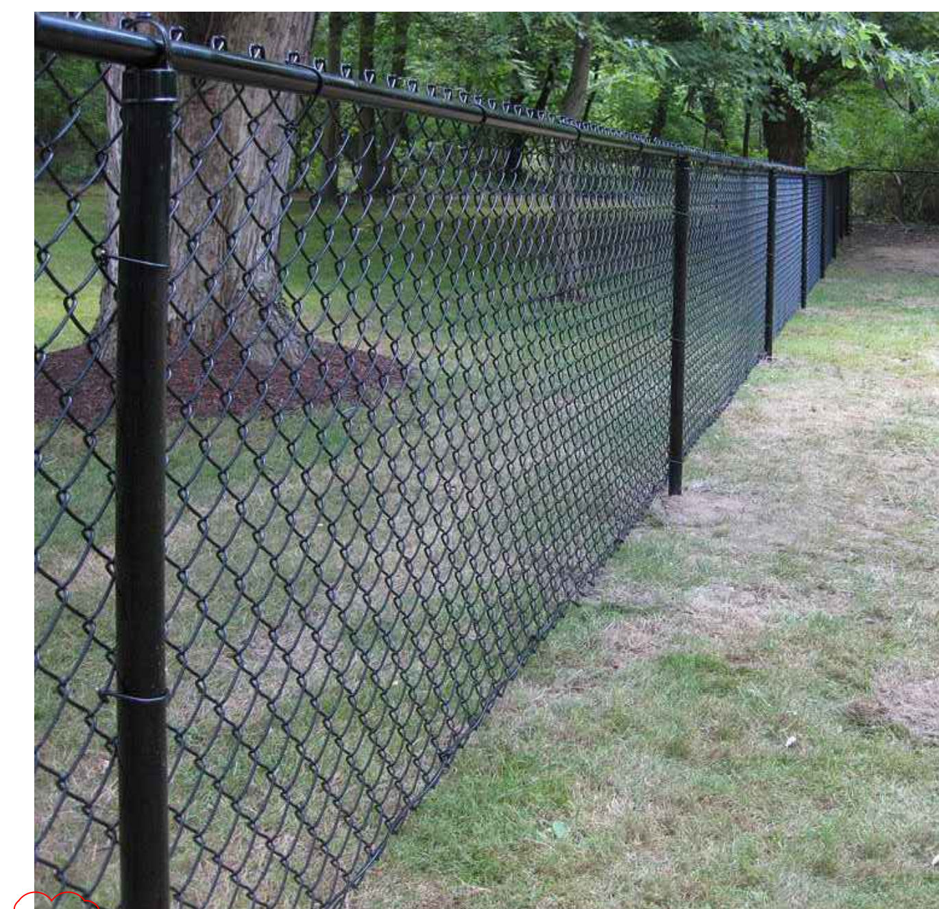
8'-0" TALL GALVANIZED CHAIN LINK FENCE FENCE FRAMING TO BE GALVANIZED 40 WEIGHT PIPE, 2.875" O.D. TERMINAL AND MAN GATE POSTS, 2.375" O.D. LINE POSTS AT 10' ON CENTER, 1.66" O.D. TOP RAIL. CHAIN LINK MESH TO BE GALVANIZED 9 GAUGE WIRE WOVEN IN STANDARD 2" MESH PATTERN. MAN GATE TO HAVE PANIC BAR WITH BACK PLATE EXPANDED METAL IN THE GATE. VERTICAL PIPES TO BE SET IN CONCRETE.
