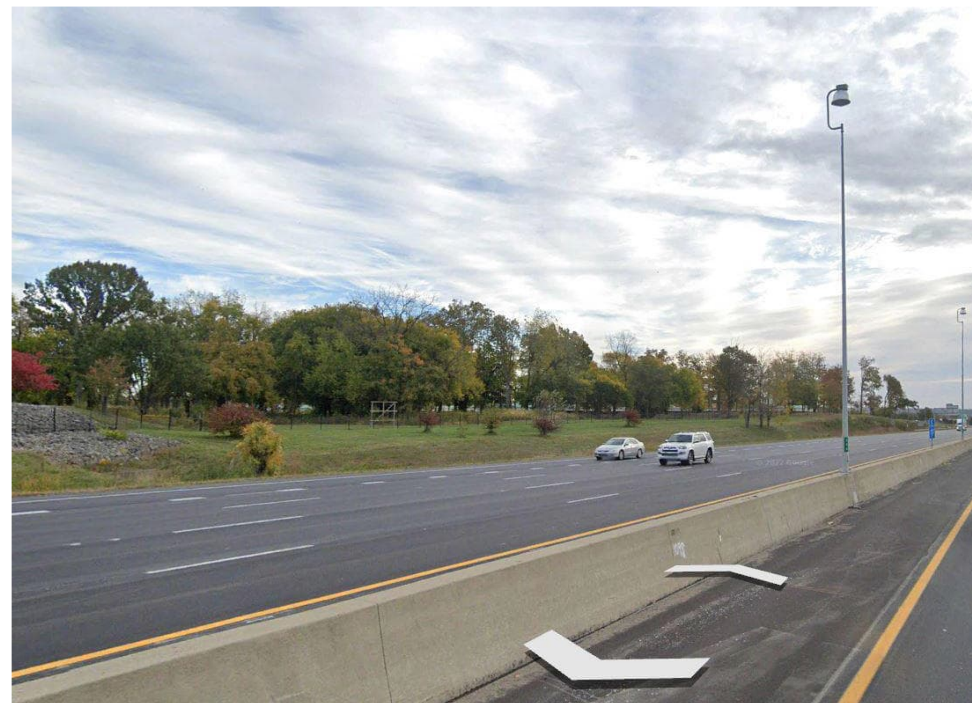
A - ACTUAL PUBLIC WAY VIEW FROM I-275 EAST BOUND
