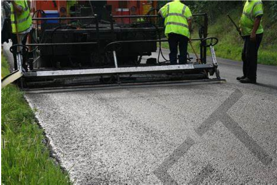
Figure 18: Typical Microsurfacing Paving Crew
