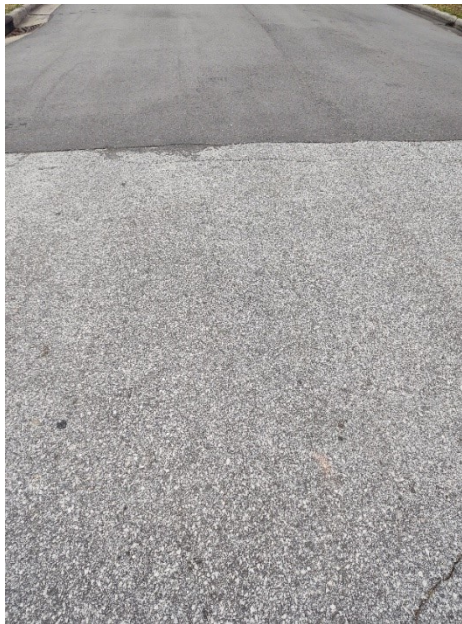
Figure 9: Oxidation versus newer pavement (top of picture)
