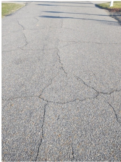
Figures 5 & 6: Block Cracking and Transverse Cracking as seen on Ocean Boulevard and Ginguite Trail
