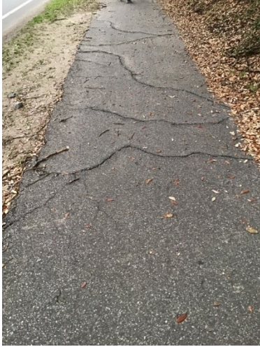
Figure C – Root intrusion cracks
