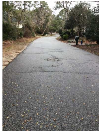
Figures 5 & 6: Block Cracking and Transverse Cracking as seen on Ocean Boulevard and Ginguite Trail
