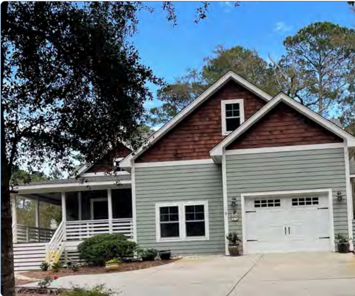
Southern Shores consists of mainly low density residences.
