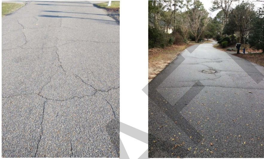
Figures 5 & 6: Block Cracking and Transverse Cracking as seen on Ocean Boulevard and Ginguite Trail
