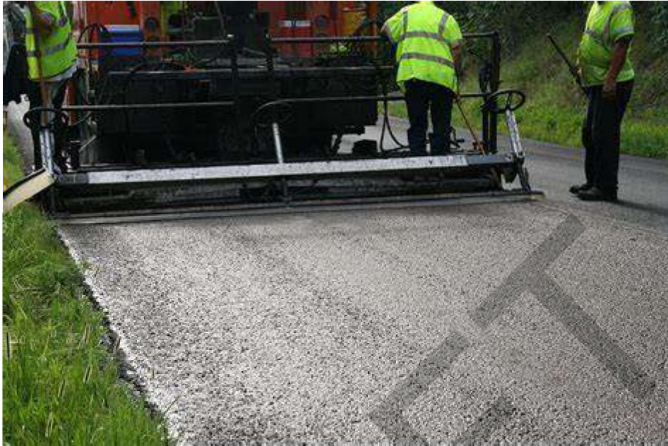
Figure 18: Typical Microsurfacing Paving Crew
