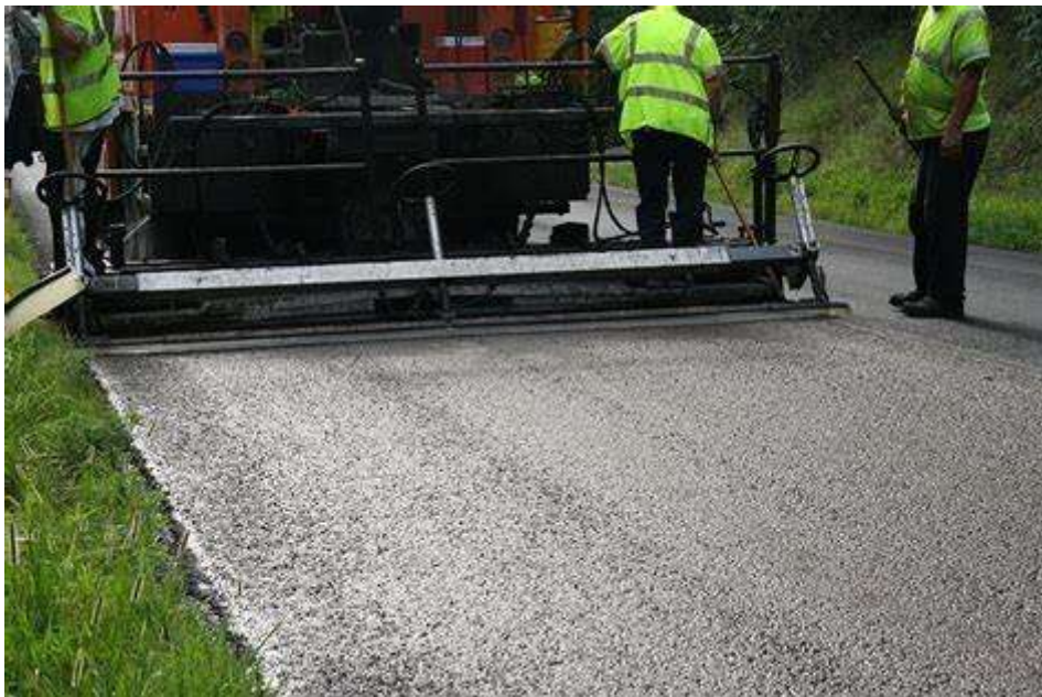
Figure 18: Typical Microsurfacing Paving Crew
