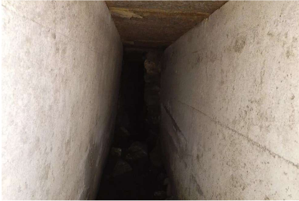
Gunite area around stone tunnel creating box culvert south of Entry 6
