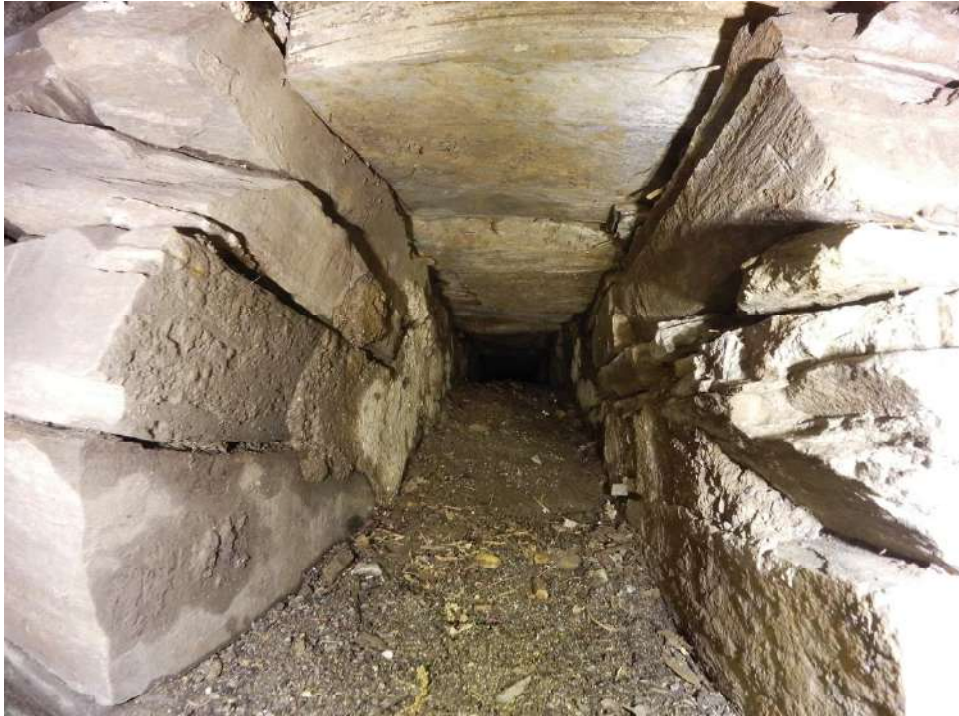
Entrance of an additional rock tunnel (1 ft x 1 ft) 2 ft from Entry 4
