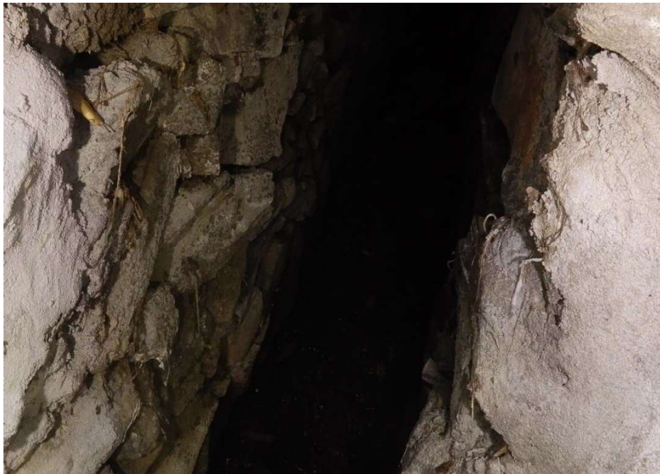
Gunite on stone wall surfaces 1 ft from Entry 8
