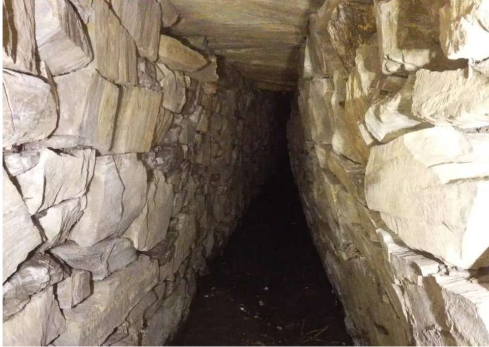
Narrow rock tunnel area 30 ft from Entry 3
