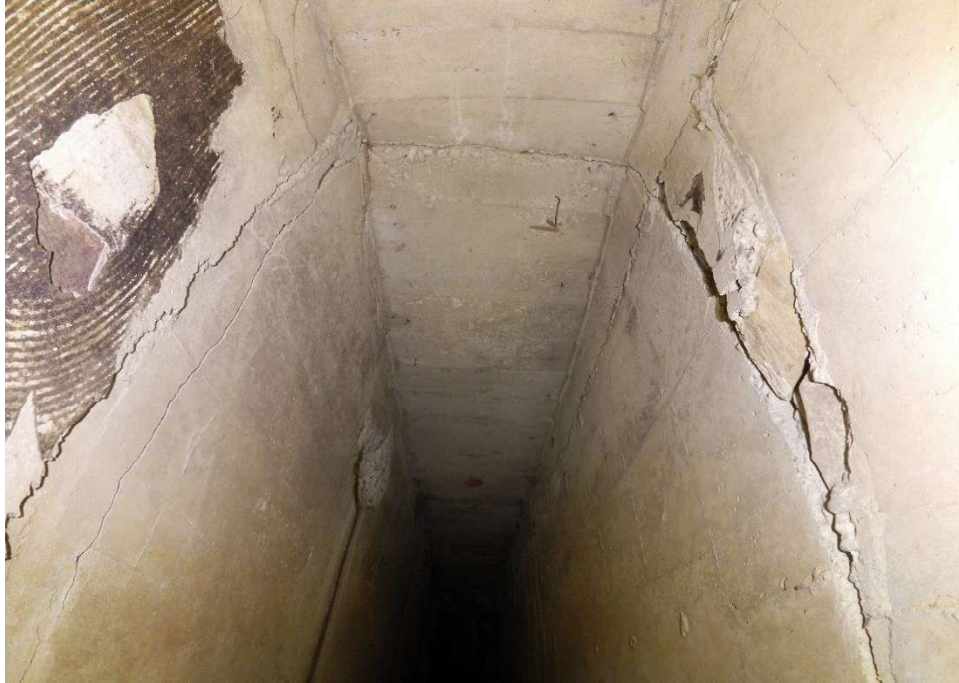
Box culvert 1 ft from Entry 10
