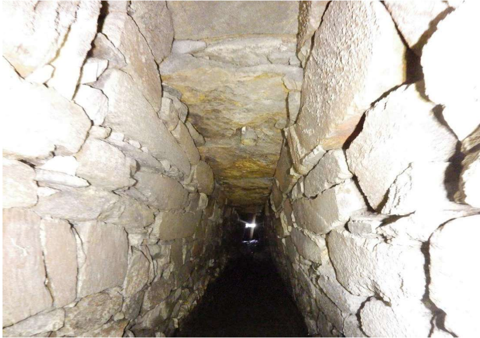
Pipe inlets on ceiling 20 ft from Entry 8
