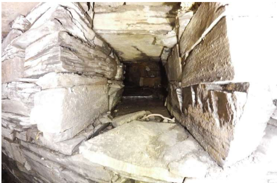
Entrance of an additional rock tunnel (1 ft x 1 ft) 2 ft from Entry 4
