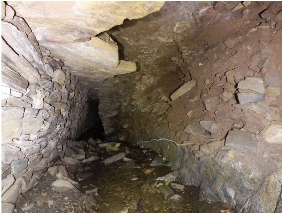
Major stone tunnel collapse 65 ft from Entry 10
