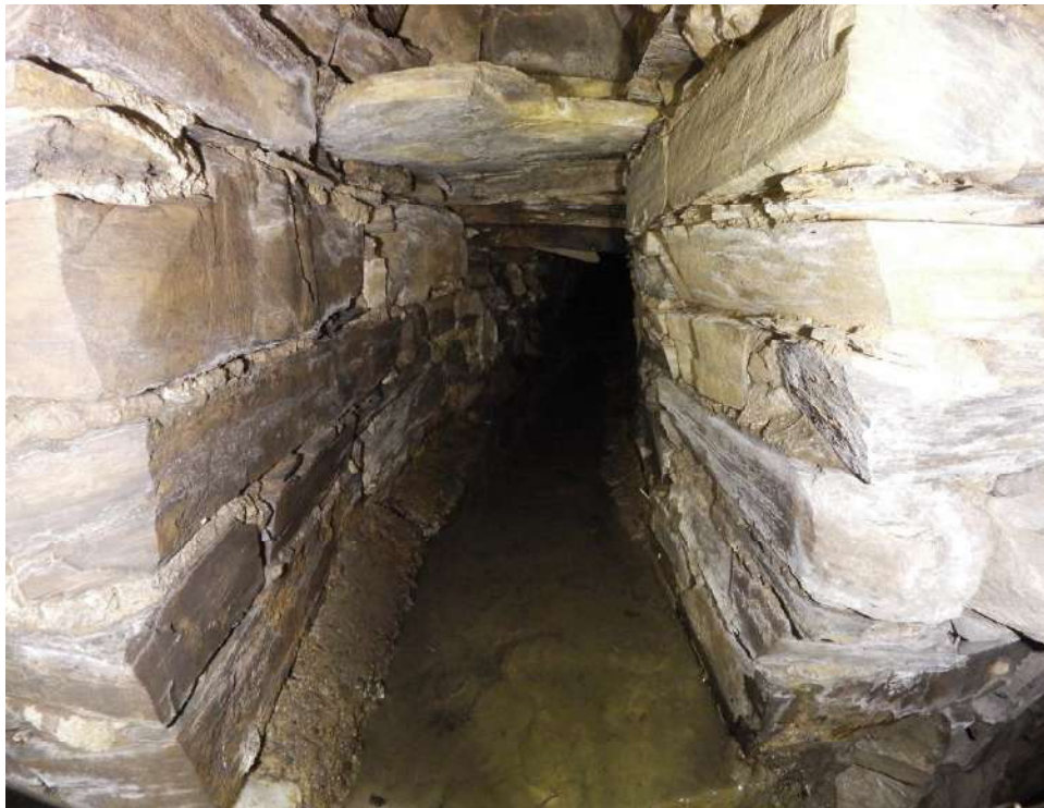
Entrance of an additional rock tunnel (1 ft x 1 ft) 12 ft from Entry 6
