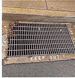
IMAGE NO. 8 DRAINAGE INLET LOOKING WESTERLY
