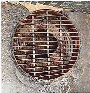
IMAGE NO. 11 DRAINAGE INLET LOOKING DOWN
