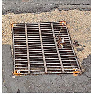
IMAGE NO. 2 DRAINAGE INLET LOOKING DOWN
