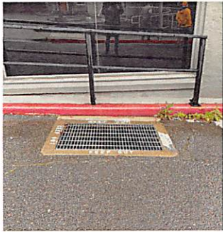
IMAGE NO. 6 DRAINAGE INLET LOOKING SOUTH EASTERLY
