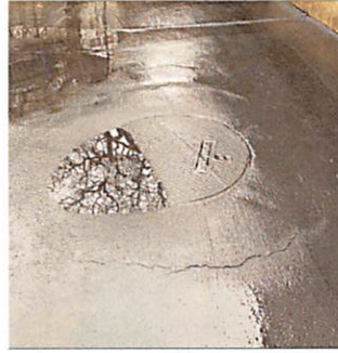
IMAGE NO. 3 STORM DRAIN MANHOLE LOOKING DOWN
