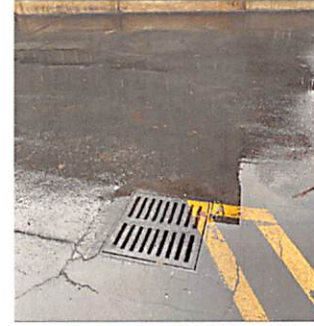
IMAGE NO. 4 DRAINAGE INLET LOOKING NORTHERLY
