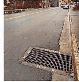
IMAGE NO. 9 DRAINAGE INLET LOOKING NORTHERLY
