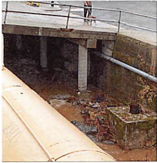
IMAGE NO. 1 CONCRETE OUTLET UNDER BRIDGE LOOKING EASTERLY
