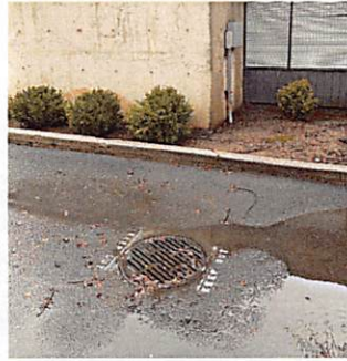
IMAGE NO. 7 STORMDRAIN MANHOLE LOOKING NORTHERLY
