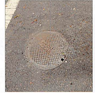
IMAGE NO. 10 STORM DRAIN MANHOLE LOOKING DOWN
