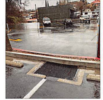
IMAGE NO. 5 DRAINAGE INLET LOOKING NORTH WESTERLY
