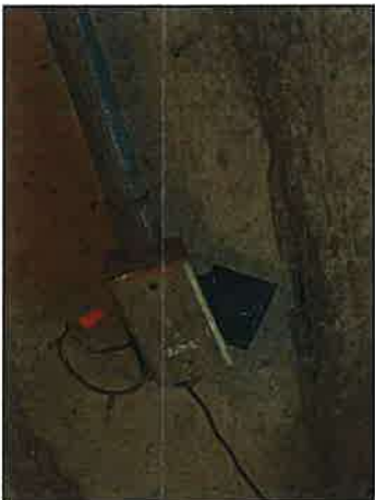
EXISTING PRESSURE TRANSMITTER JUNCTION BOX
