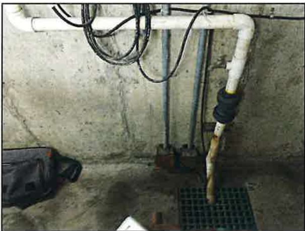
EXISTING FLOOD SWITCHES AND SUMP.
