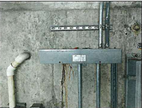
EXISTING FLOOD SWITCH JUNCTION BOX
