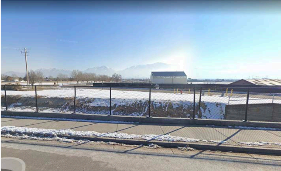
Example of concrete sidewalk with fence and curb and gutter
