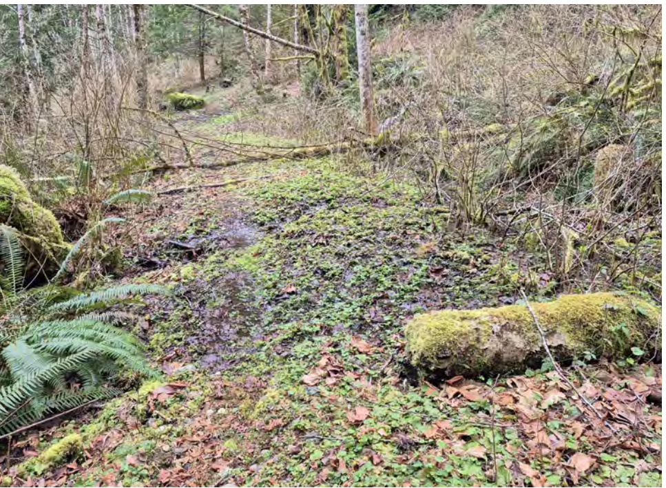
PHOTO5: Ponding upslope of embankment and flow of water over embankment near culverts at STA 49+50 resulting in minor trail erosion. View to the west.
