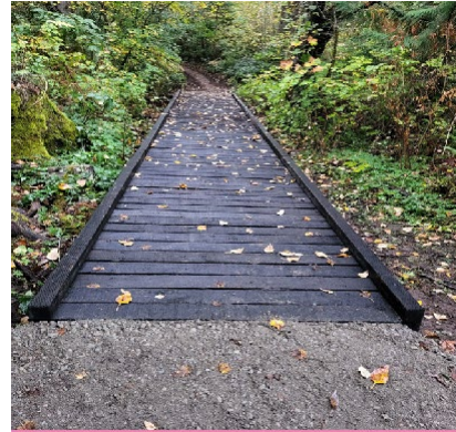
Steller Boardwalk Replaced
