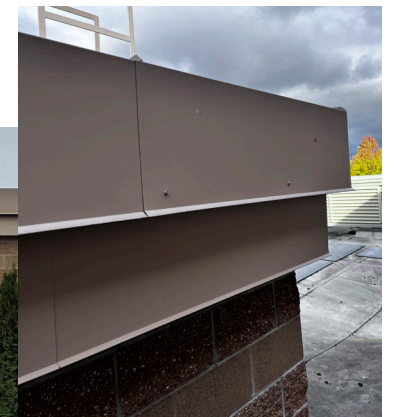
Parapet Color & Detail
