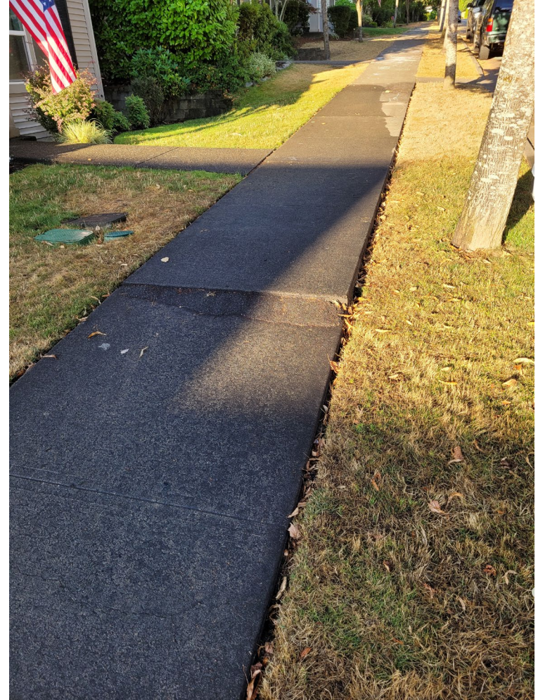
Cold Mix Asphalt
