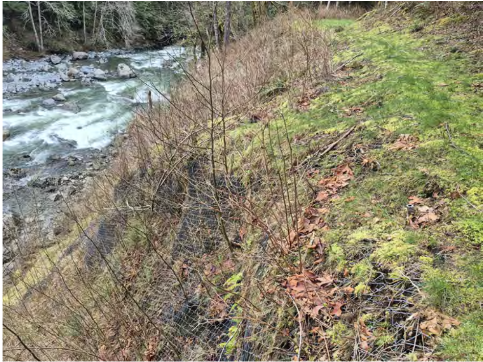
PHOTO 4: Landslide headscarp downslope of the pipeline. Orange flag is AMP-04, STA 41+80. Pipeline is in upper part of photograh, about 11 feet from head scarp.
