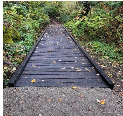
Steller Boardwalk Replaced
