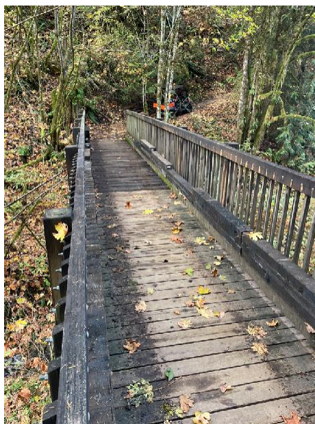
Deep Creek Bridge Deck Partially (left) and Fully (above) Replaced
