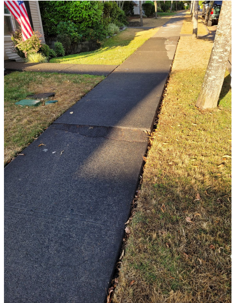
Cold Mix Asphalt
