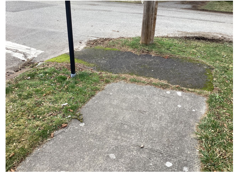
No Detectable Warning Surface
