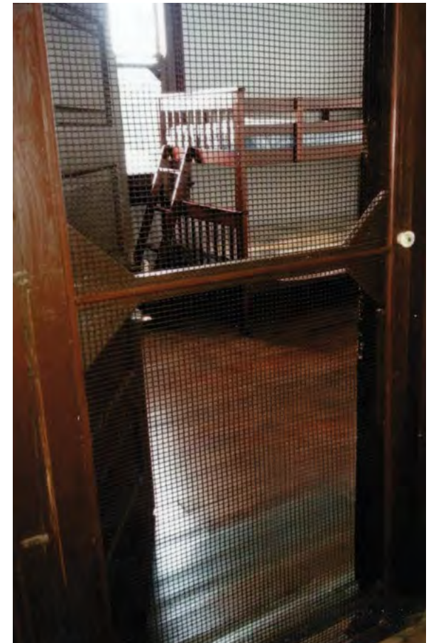
[31] An interior screen door at the entrance to individual apartments is a historic feature traditionally used to help circulate air throughout the building.
