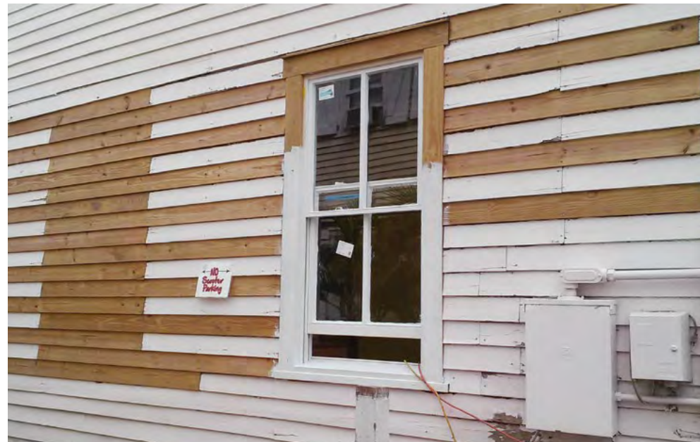
[8] Rotted clapboards have been replaced selectively with new wood siding to match the originals.
