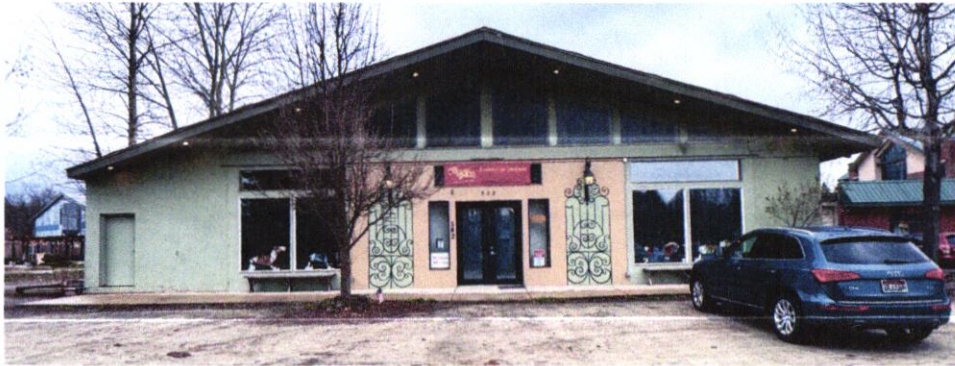
South Face - Leftside with decorative painting
