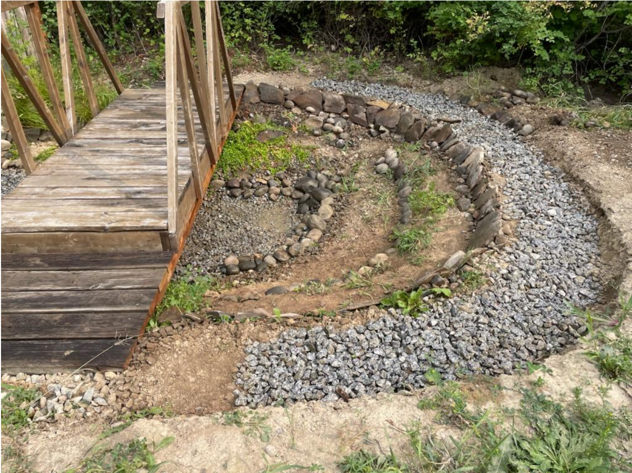
Drainage Ditch – End has been excavated and landscaped
