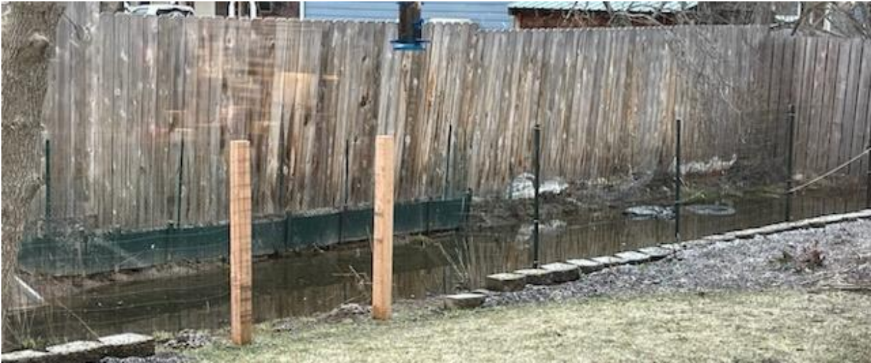
Drainage Ditch - Backyard
