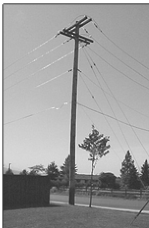
Figure 7: Incorrect planting
