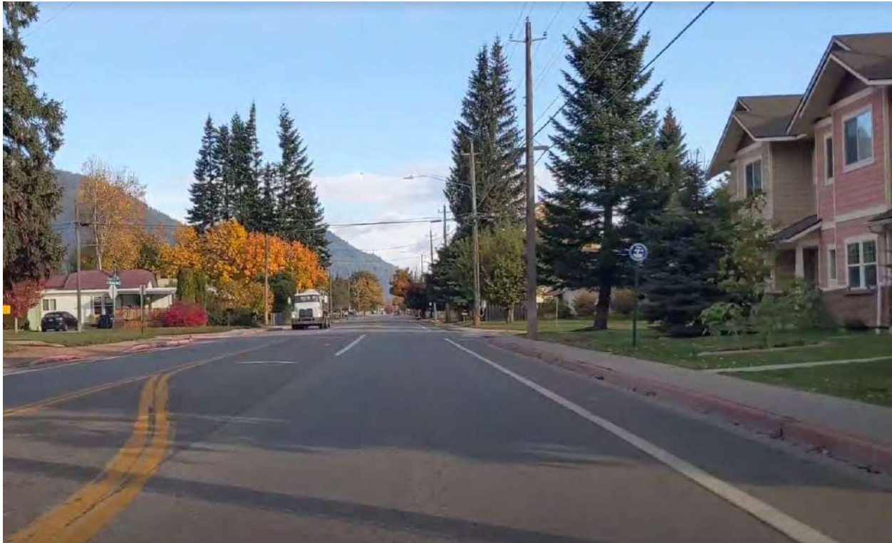
Observation 8: Substandard bus stop (Photo: Fehr & Peers).
