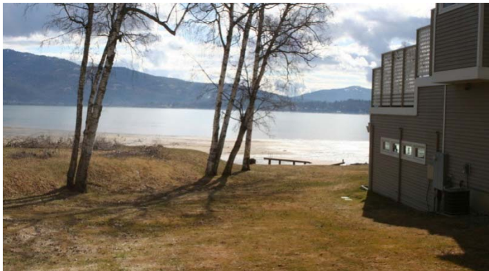
Figure 20. Panoramic photograph of Ella right-of-way
