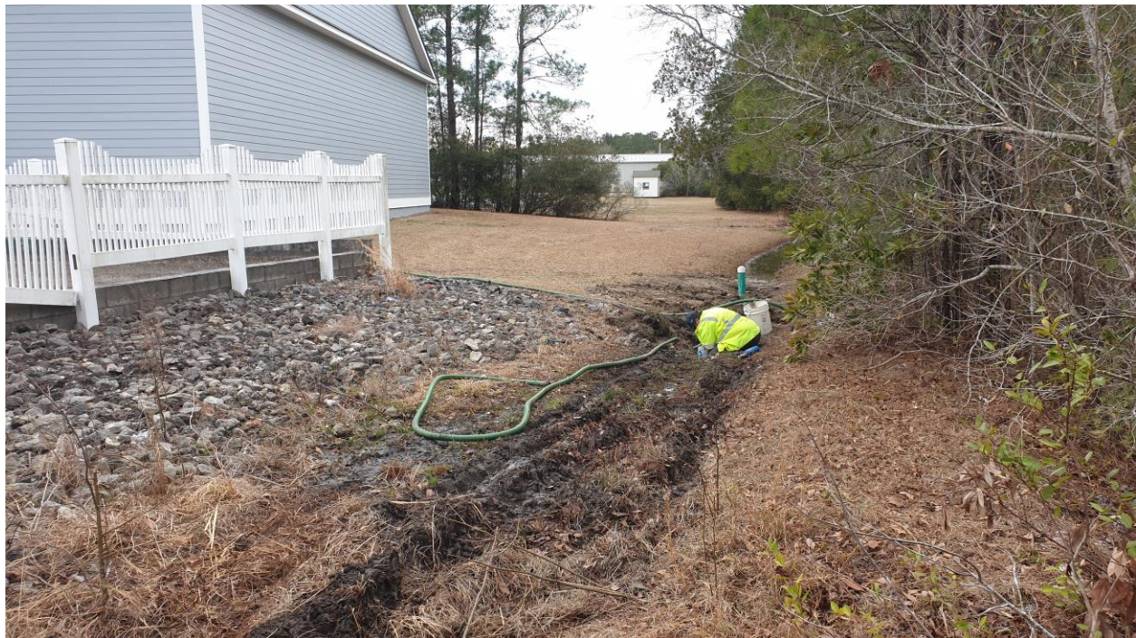
Gravity Sewer Repair
