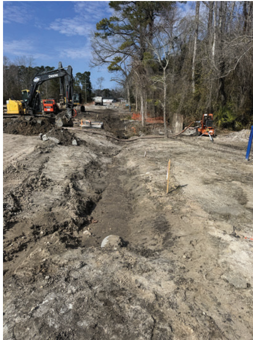
(P1) South end of wall
