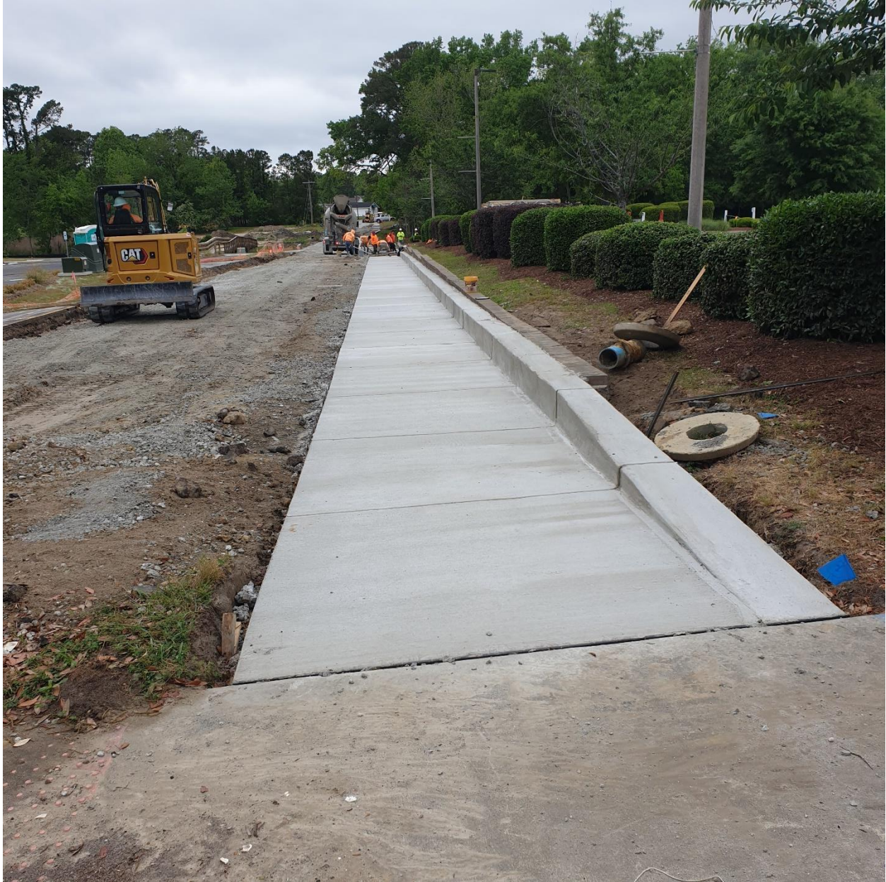
New sidewalk on Mulberry St.
