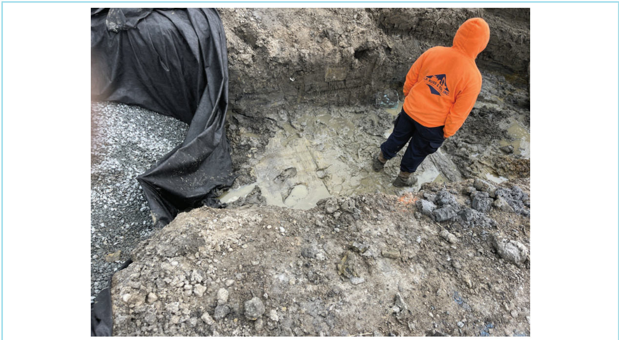
(P2) South end of Northwest retaining wall
