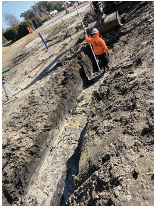
(P2) South end of Northwest retaining wall
