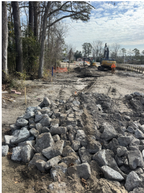
(P2) North end of wall
