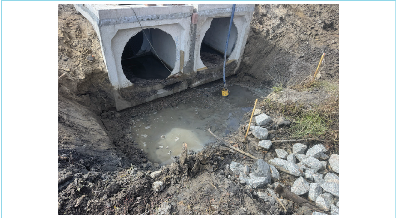
(P4) Footing on arrival
