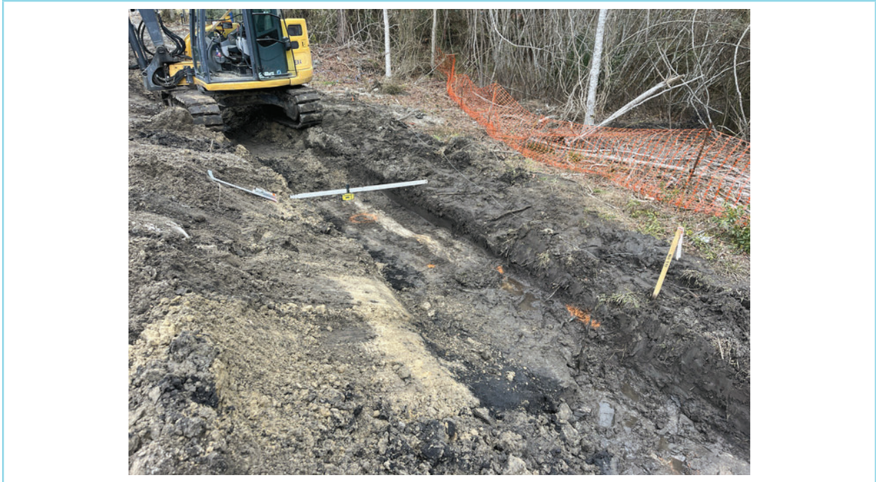
(P1) North end of Northwest retaining wall
