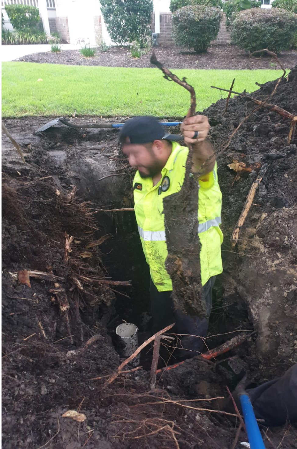
Root Removal From Gravity Sewer Service
