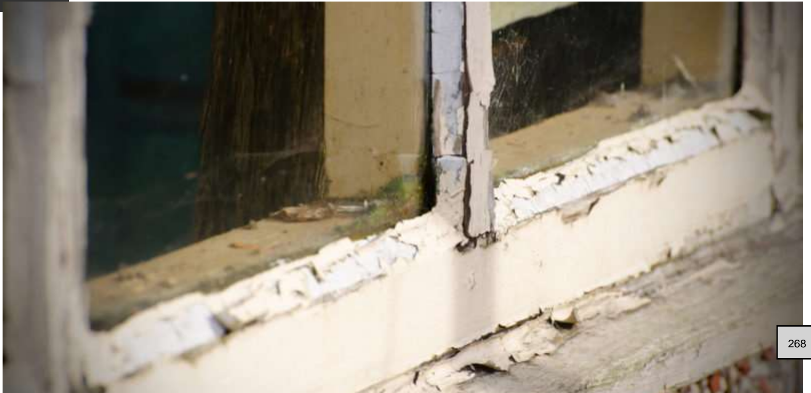
Lead-Based Paint on Windows
