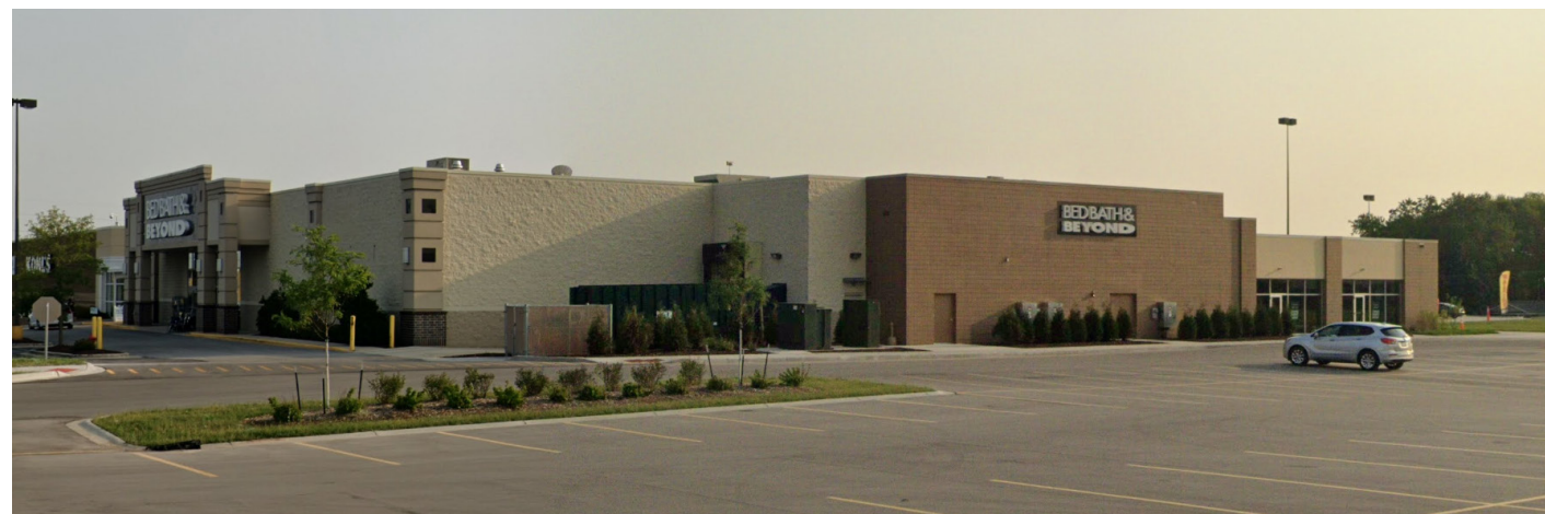
Existing North Elevation (Side) No work, existing to remain
