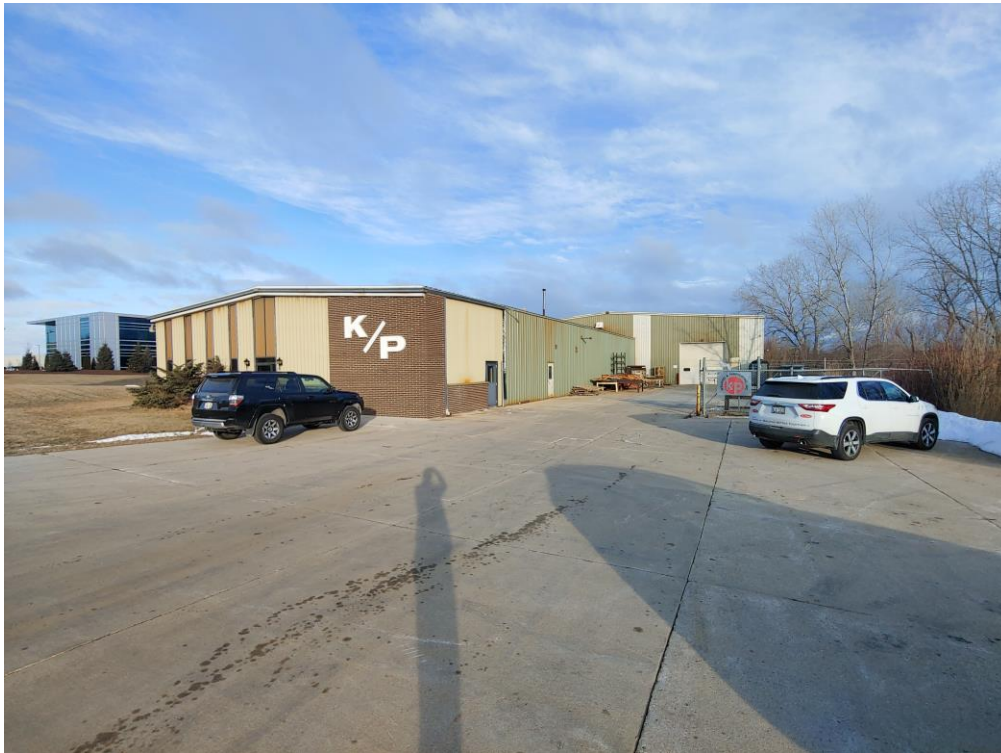
Existing west elevation at entry
