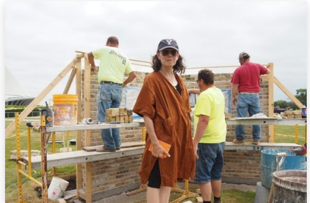
Hamilton on site during the Milwaukee build, working with the masonry crew.
