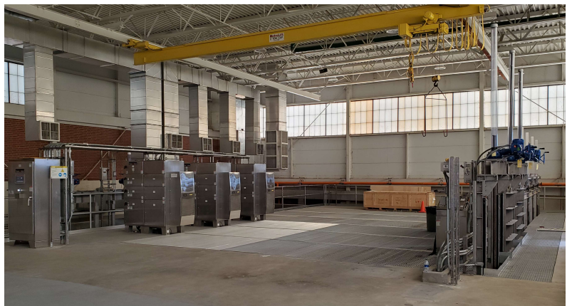
New Trojan UV Disinfection System – MMSD.
